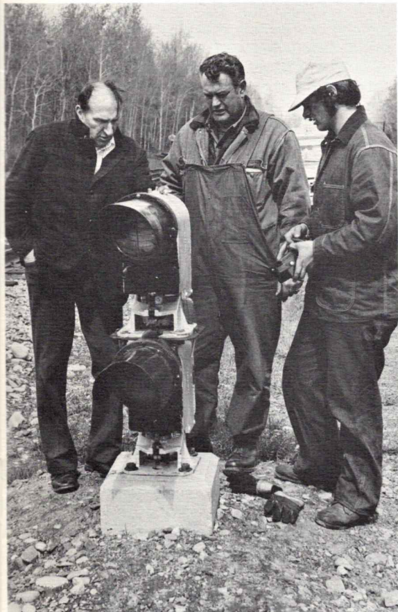
Herbert Sullivan, signal supervisor, left; R.H. Sawyer, center, signal foreman; and J.P. Cavet, signal helper, test signal at Canaan.
