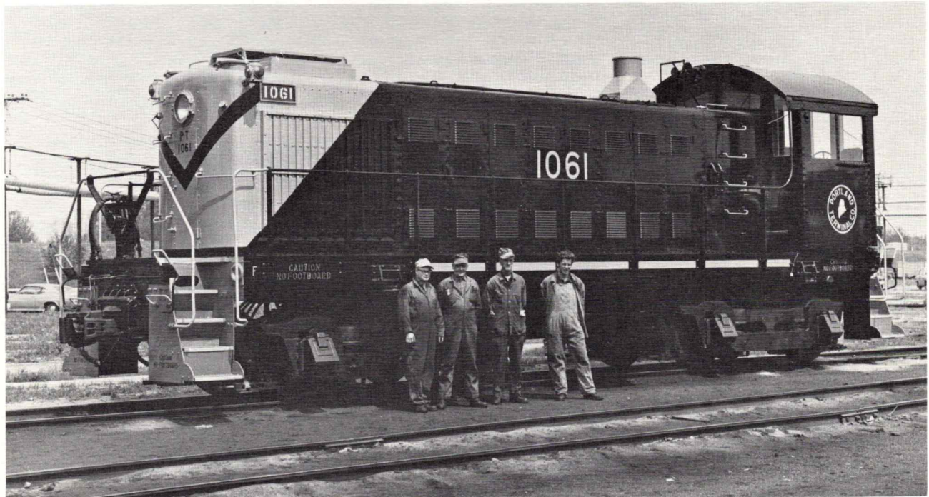
Portland Terminal number 1061 is shown after a complete overhaul by Portland Terminal forces. The new Federal Railroad Administration switching step should be noted. Left to right: Oley Kline, electrician; Joe Fontaine, electrician; Ernie MacVane, machinist; and Harry Lawrence, machinist. Also involved was Frank Blair, electrician, who was unavailable for this photo.
