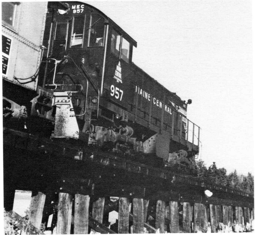
The last train into Eastport moves slowly over the 222-foot pile trestle at Pennamaquan in Pembroke on Maine Central's 16-mile Eastport Branch. Photo by Herb Cleaves.
