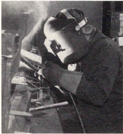
Welding requires a sturdy welding hood with a special lens to prevent "welding flash burn" to the eyes. Al McCann at Rigby Enginehouse wears such a hood.
