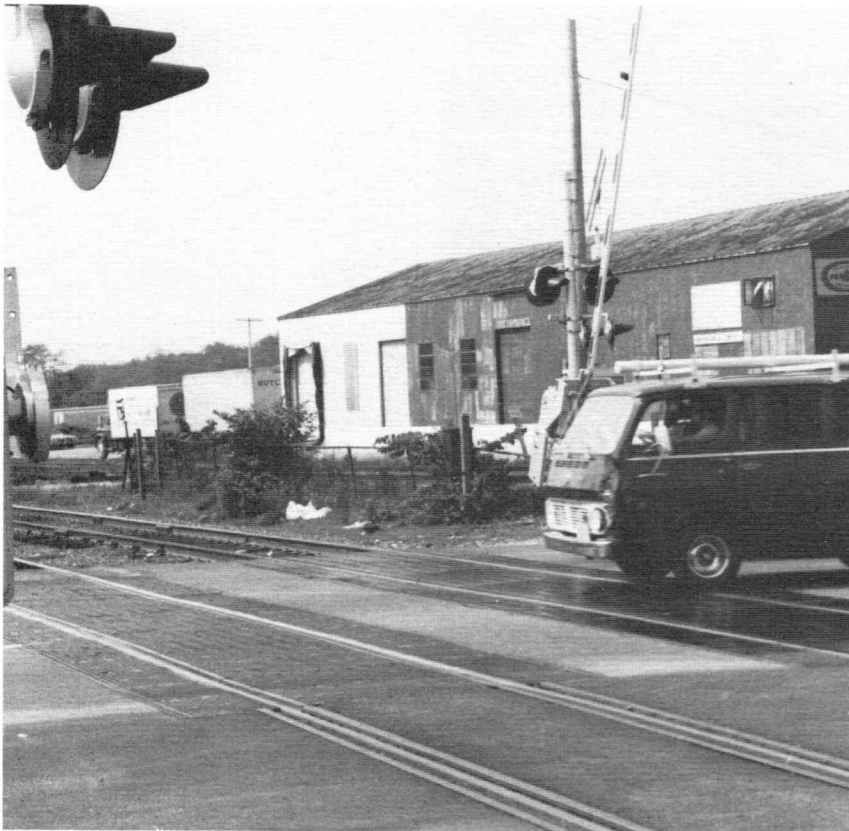
The new rubberized crossing at Congress Street in Portland. A van—with lights flashing, the warning bells ringing and the gate coming down, rushes to beat the train.
