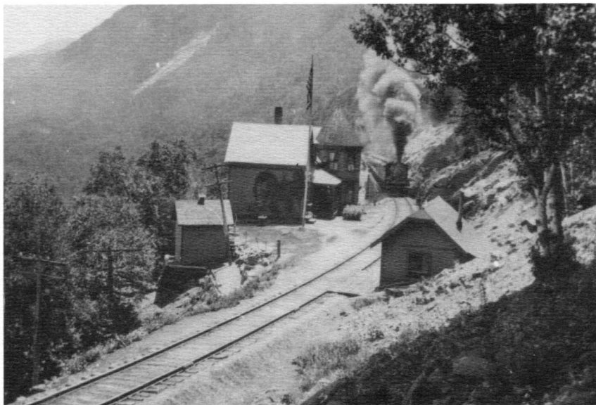
Although this picture was taken a few years after WW 1, the section house in the Notch looked about like this in 1917, when Mr. Leavitt was assigned there as a guard. The locomotive is of the 400 series, built in 1918. (Photo courtesy Ray Evans)
