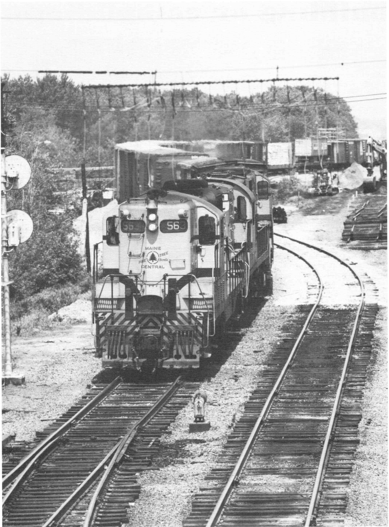
Maine Central's BR-4 negotiates the new shoo-fly around the Broadway underpass bridge. It was one of the first trains to pass over the new section of track. (Ron Johnson photo)
