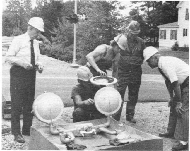
Another stop on the Spring Cleanup inspection itinerary was at North Conway, where the officials watched progress on a signal modernization project. From left, A.J. Travis, executive vice president; Andy Cash, assistant signalman; Rusty Fearon, signal helper; Ray Sawyer, foreman; and John F. Gerity, MEC president.
